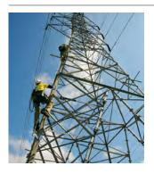
Flexible enough to accommodate every safety need for working at height, Latchways vertical systems are ideal for personnel accessing high-voltage transmission towers or transformers in substations.
