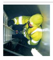
When ascending a ladder within a new build or retrofit turbine, rely on MSA Latchways TowerLatch to deliver the ideal hands-free solution, securing the climber to the cable via the chest D-ring on their full-body harness.
