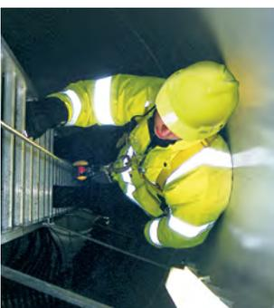
When ascending a ladder within a new build or retrofit turbine, rely on MSA Latchways TowerLatch to deliver the ideal hands-free solution, securing the climber to the cable via the chest D-ring on their full-body harness.
